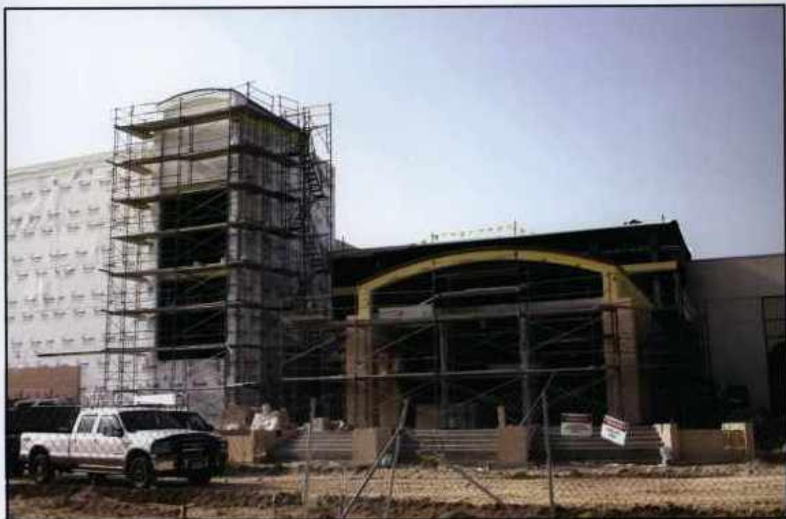
Construction of the new West Pasco Judicial Center continued during 2005.
